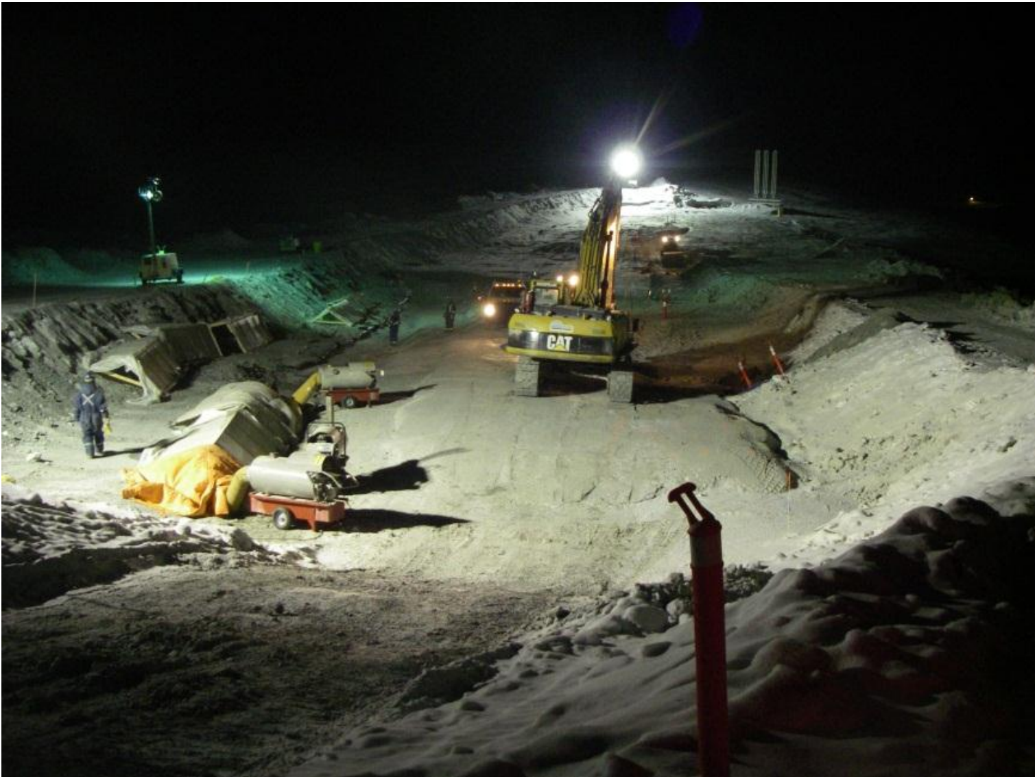
Photo 7: Cleanup of the frozen core placed on Feb. 12. On the left side of the photo laborers are removing 5/8 crush from the GCL liner.
