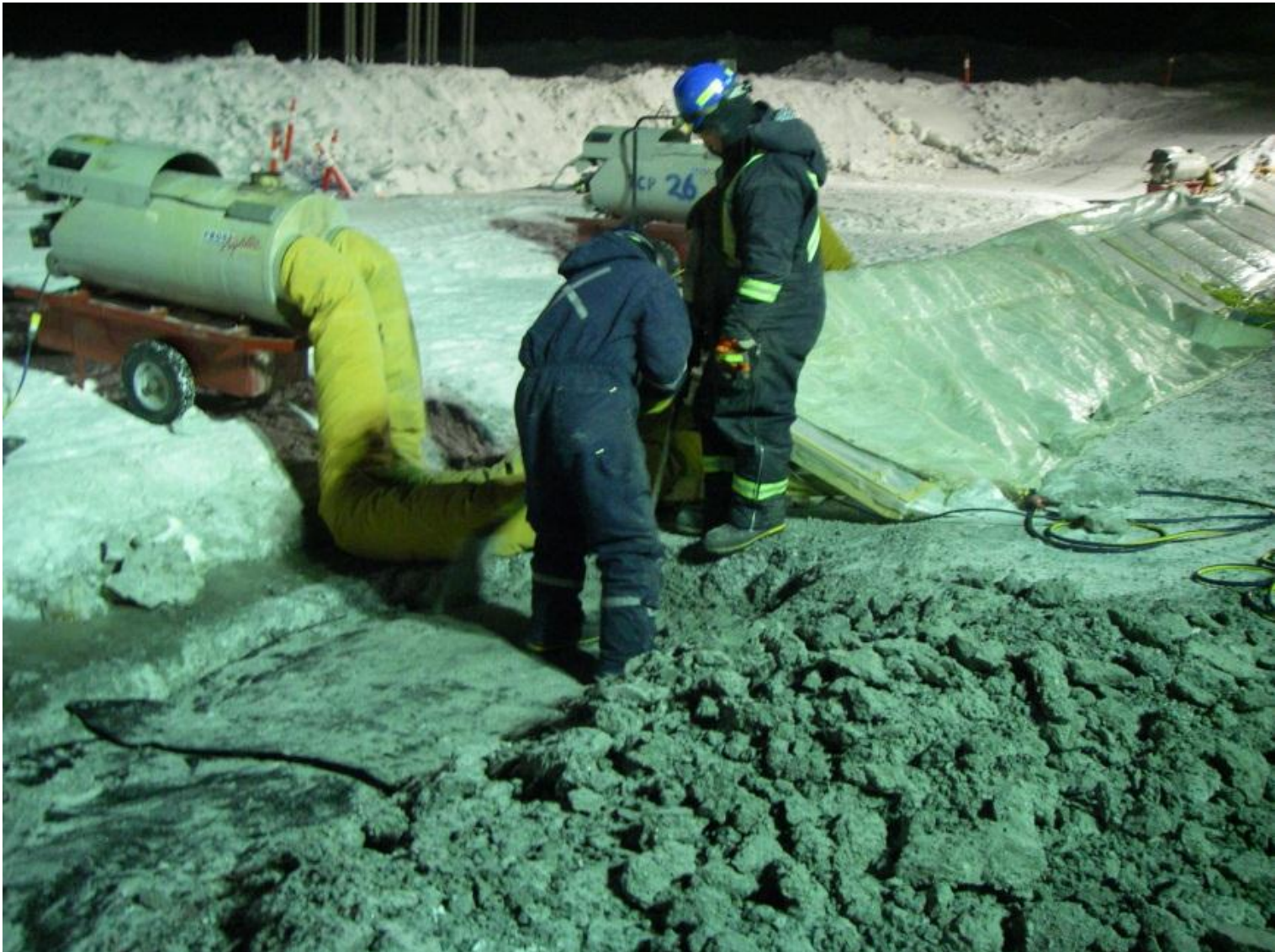
Photo 6: Laborers breaking up the frozen 5/8 crush using a jack hammer.
